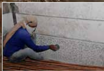
Soft cleaning of ornamental motifs and plasterwork
