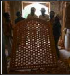
Installing sandstone lattice screens
