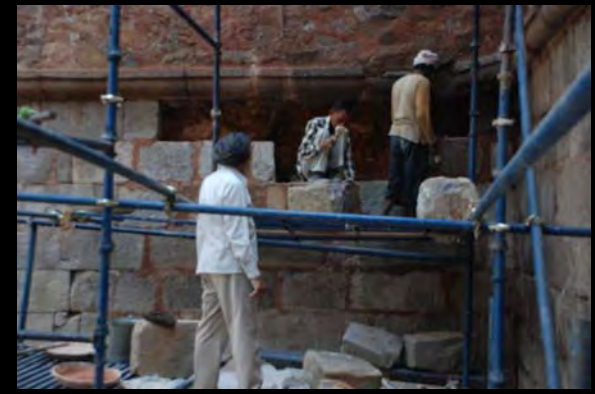
Collapsed stone masonry was reconstructed following the existing profile and original construction technique.
