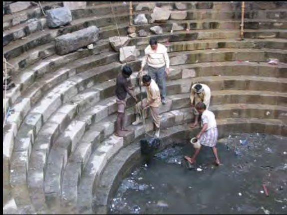
Masonry Stones which had fallen in the Baoli and were buried in the sludge were manually collected washed and dressed again before reuse in the masonry
