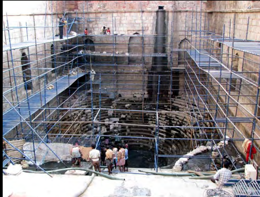
Heavy stones were lifted by cranes to the wall height for repair works, February 2009
