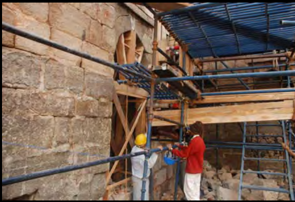
Temporary supports were provided on structurally weak arches and wall for safe working conditions
