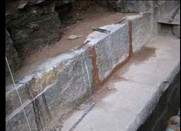
Stone members joined together using copper dowels. Ashlars masonry wall fixed with the back fill using stone slabs
