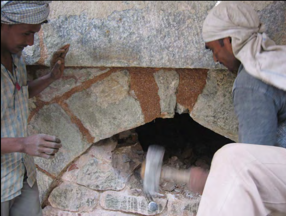
Stone craftsmen are opening the closed arch passage on east wall. April 2009
