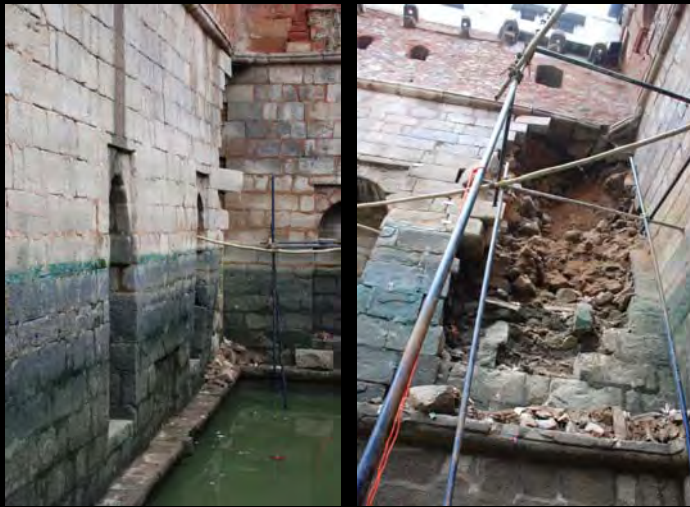
Collapsed eastern wall of the Baoli, July 2008
