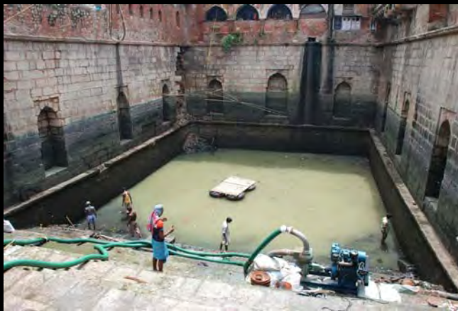
Water of the Baoli was drained out regularly to maintain the water level required for repair works
