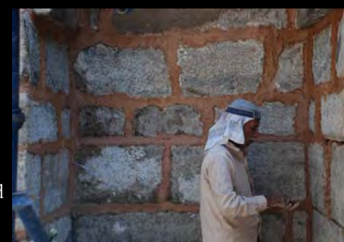
Repointing of the stone masonry with lime mortar March 2009
