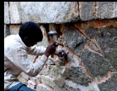
Removal of 2-3 cm thick epoxy layers March 2009
