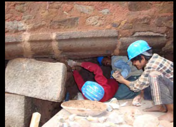
Stone masons reconstruct the top layer of the Baoli wall
