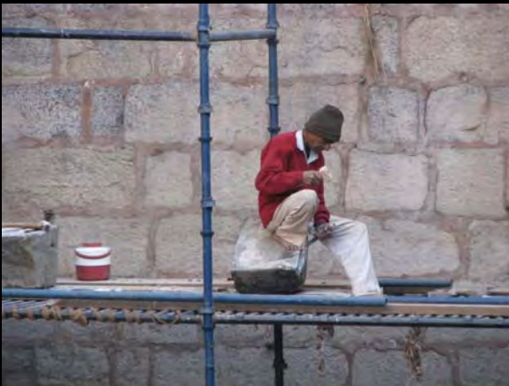
Masonry Stones were dressed on site using hand tools
