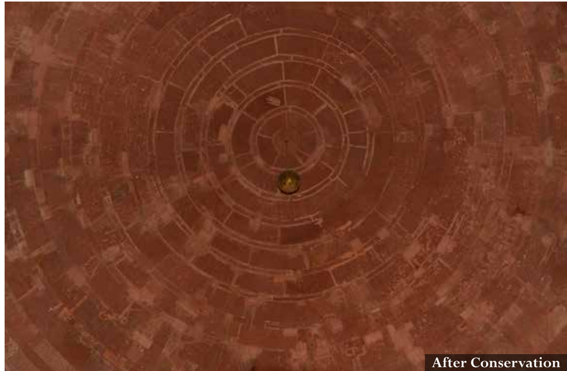
Photograph showing layer of acrylic paint on the internal surface of the dome
