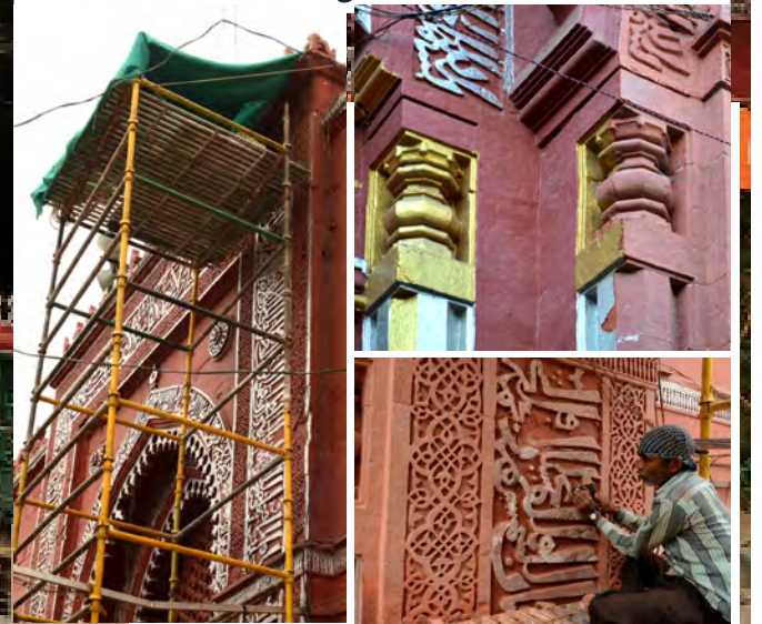
FACADE: During Conservation
