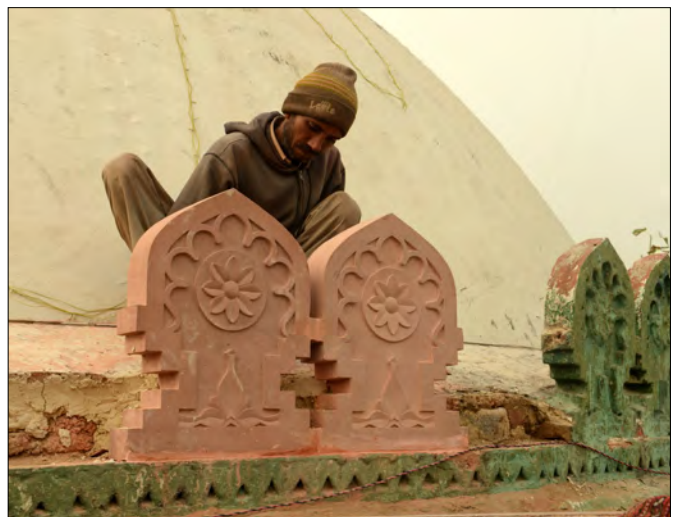
Conservation works at the 14 th century Khilji mosque required scrapping of several dozen paint and cement layers prior to repair or replacement of the damaged sandstone elements.
