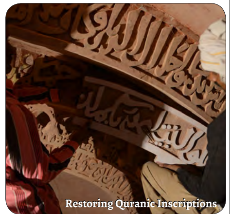
Removal of multiple layers of lead paint
