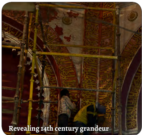
Removal of multiple layers of lead paint
