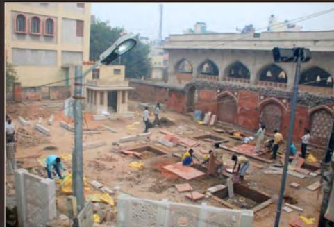
The iron fencing of Mirza Ghalib's tomb enclosure is being replaced with a stone masonry wall with sandstone lattice screens that will help create a courtyard effect and also lend considerable historic character to the principal street leading to the Dargah
