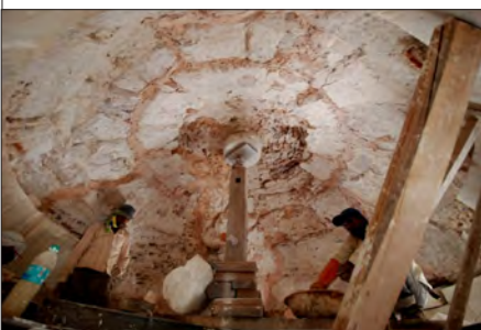
▲ Stone carvers fix the repaired marble elements back to their original location on the structure
