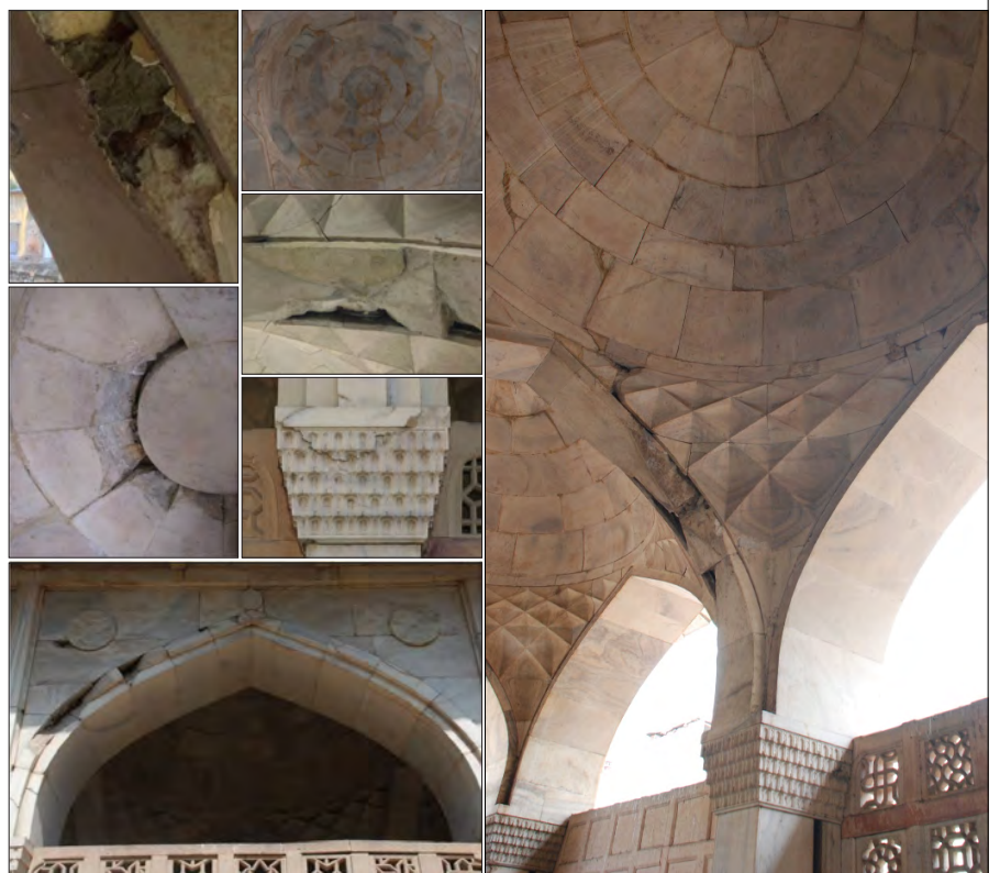
Material Deterioration due to past repairs in white cement – masking the damage but allowing the deterioration to accelerate; Chipping of Marble elements like domes, arches, facade, pendentive, jaalis and column capitals; Rusting of iron dowel due to water seepage led to bursting of the marble
