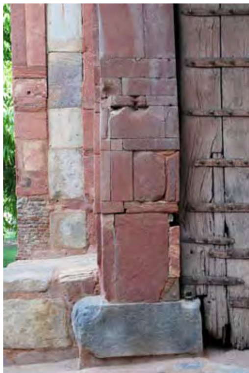
(Right) Following a stone-by-stone documentation, decayed sandstone was replaced by new stone pieces by carefully matching the original.
