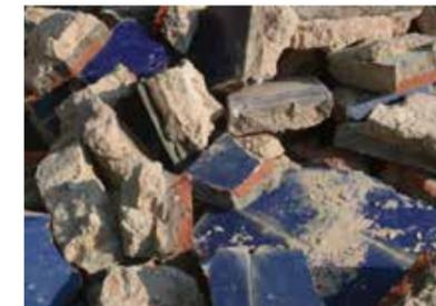
*(Below) Removal of tiles installed on the dome and drum of Sabz Burj in 1986 and the cement layers.*
