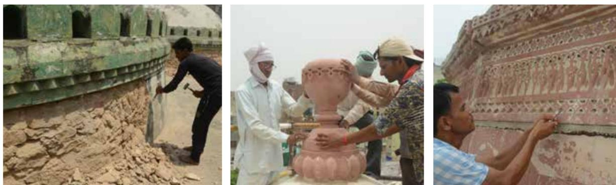
(Above) Dismantling of the cement plaster from the drum of the dome; Restoration work of the finial made in red sandstone; Careful removal of multiple layers of the paints from the ornamentation work of the dome in red sandstone.
