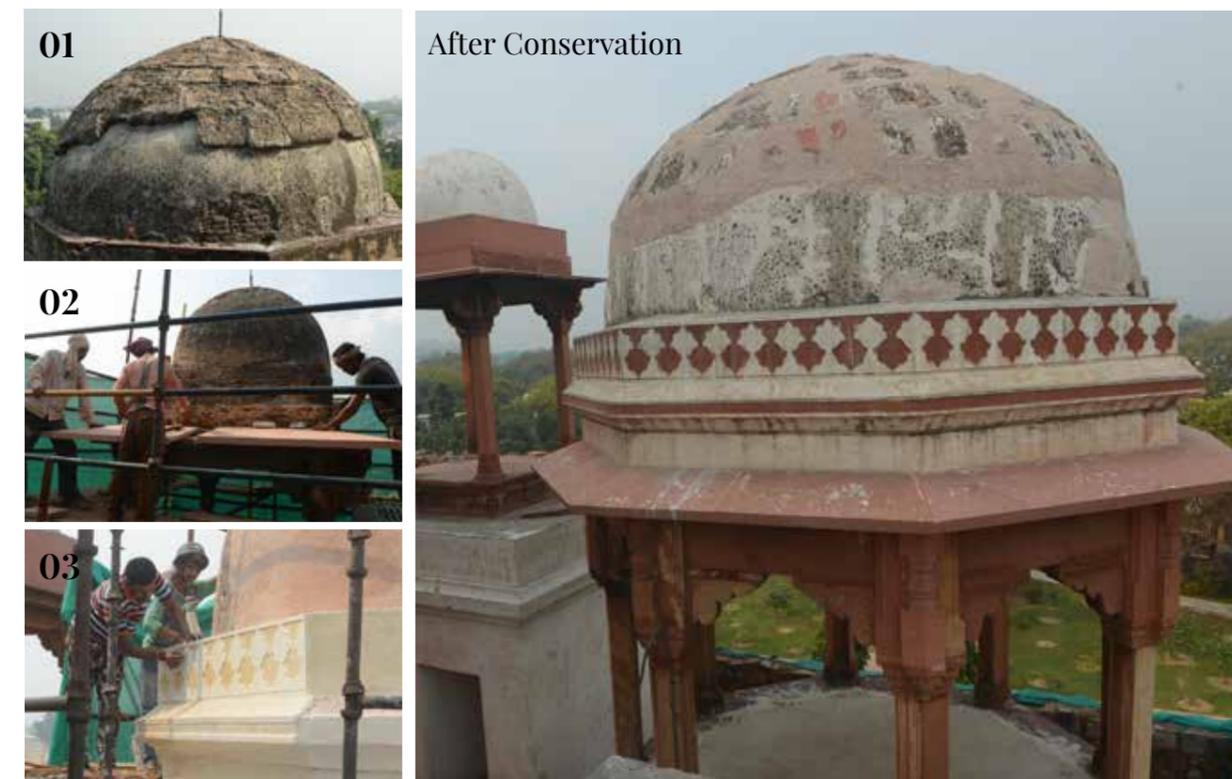
(Left column images) As with other portions of the structure, the four corner canopies were covered with cement layers, these have been renewed, the cracks repaired with traditional lime mortar; (Right) After conservation view of the canopy after removal of cement and restoring the fallen chajjas/eaves.
