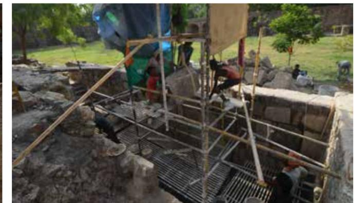
*Desilting of accumulated rubble was also carried out, leading to the re-opening of groundwater aquifers.*
