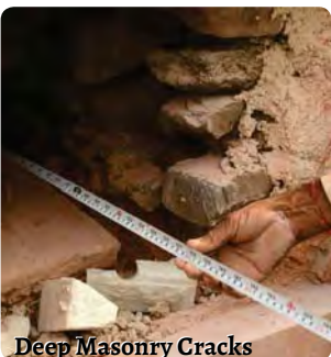
Deep Masonry Cracks
