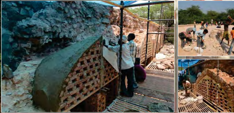
Introducing traditional materials and techniques in masonry
