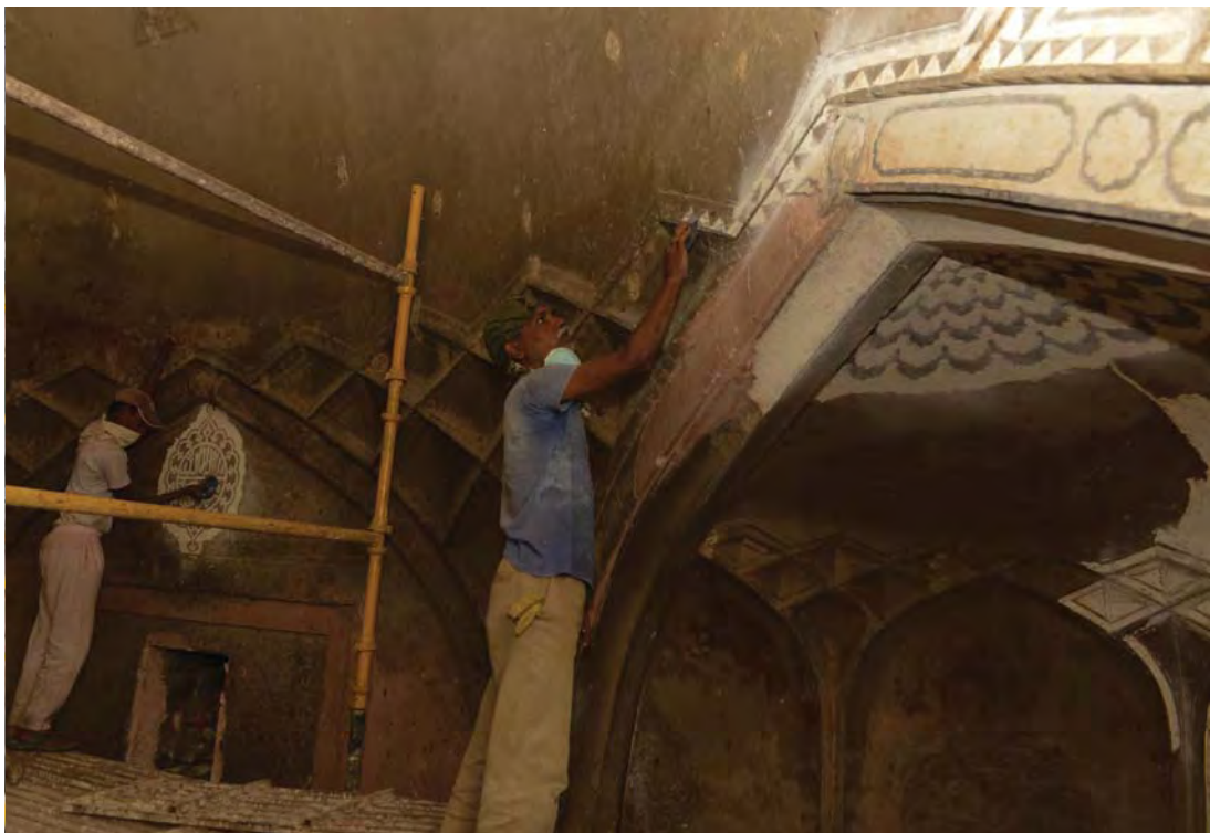
(Above) View of the main tomb chamber before conservation, when it was covered in soot, paint, and limewash; (Below) Main Tomb Chamber during conservation, where the walls and alcoves were cleaned using soft brushes and water.
