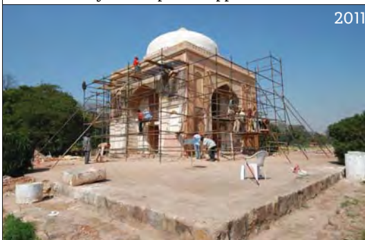
Removal of cement plaster applied in 2003-07
