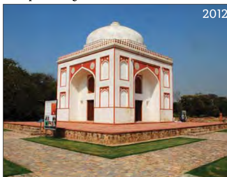
Replastering in lime mortar in 2012
