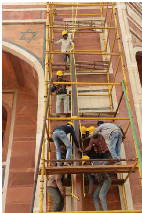
(Right) The 22 feet tall tree log being manually lifted to the dome of Humayun's Tomb. Since a significant portion of the wooden shaft was embedded in the dome masonry a tree log of 22 feet height was procured and carved to the original octagonal profile. In order to prevent repeated snapping, the base of the log was encased in a thin sheet of copper up till the top of the dome.
