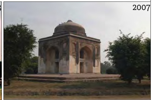
2003 repairs disintegrated, requiring second phase of cement repairs
