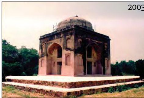
Cement repairs undertaken in 2003
