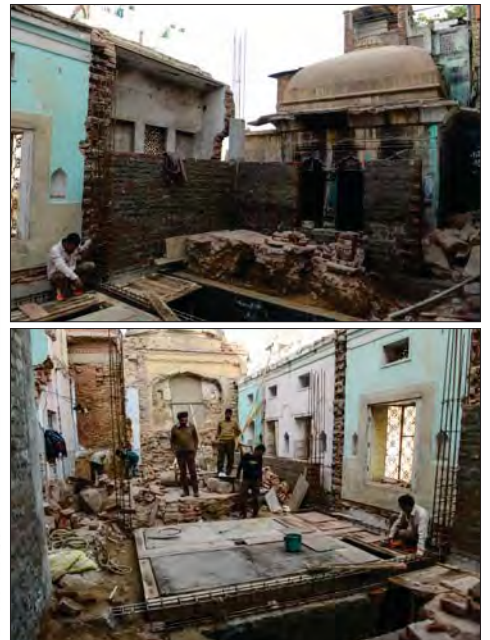
Work underway to reconstruct the Baoli arcade. This required the modern structure to be demolished and rebuilt 3 feet inside.
