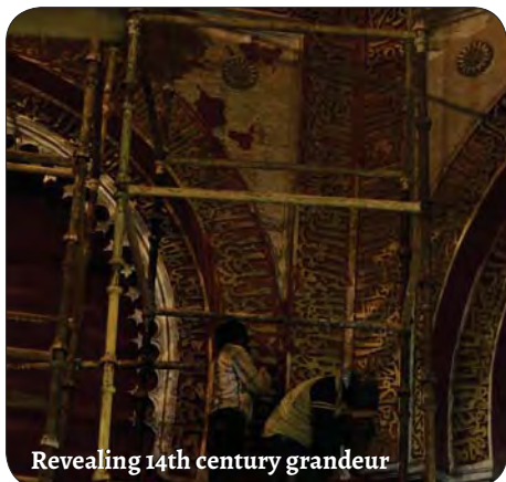
Removal of multiple layers of lead paint
