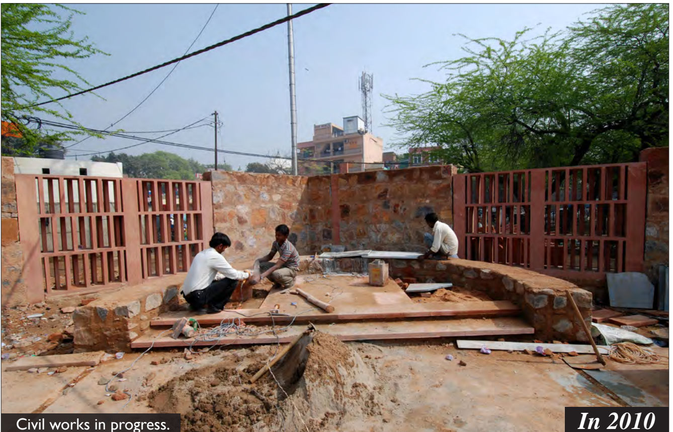
Construction of Stone Jalis along boundary wall.
