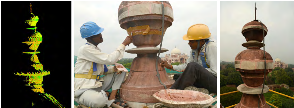
(Left) Finial of Nila Gumbad- Image generated using 3-D laser scanning Data (Centre) Craftsmen restoring the stone finial which is at the height (Right) Finial restored
