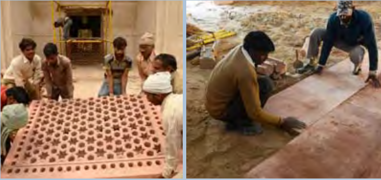
Reinstalling Sandstone jaalis and paving
