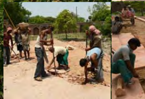
Removing cement concrete from terrace, plinth and main hall
