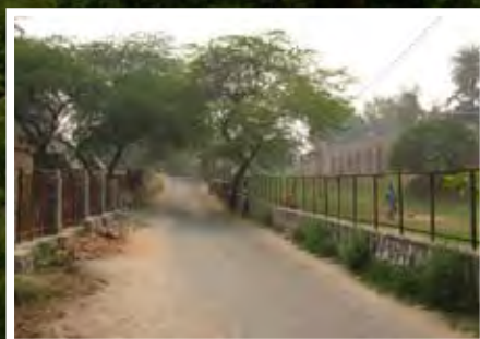
Shifting of Road
